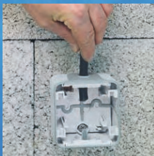
2/ Insert the cable through the end cap
