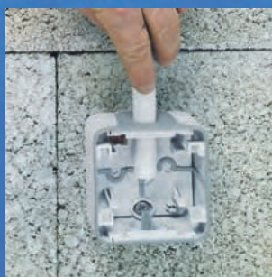
2/ Insert the tube through the end cap
