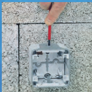
1/ Pierce the end cap using a screwdriver
