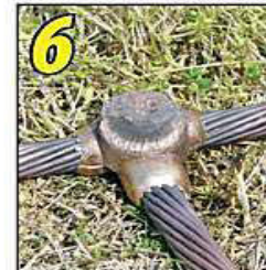
6 Remove weld and clean mold before making next connection.
