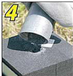
4 Place a small amount of starting powder in the ignition pocket.
