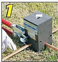
1 Position cleaned conductors in mold.
